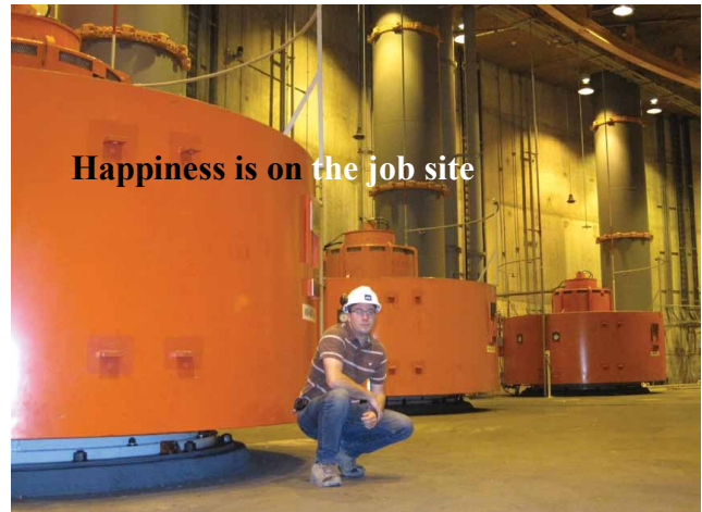
Engineer Alexandre Frigon in front of synchronous engines of 5,000 horsepower to 4.6 kilovolts at the sewage treatment plant.
